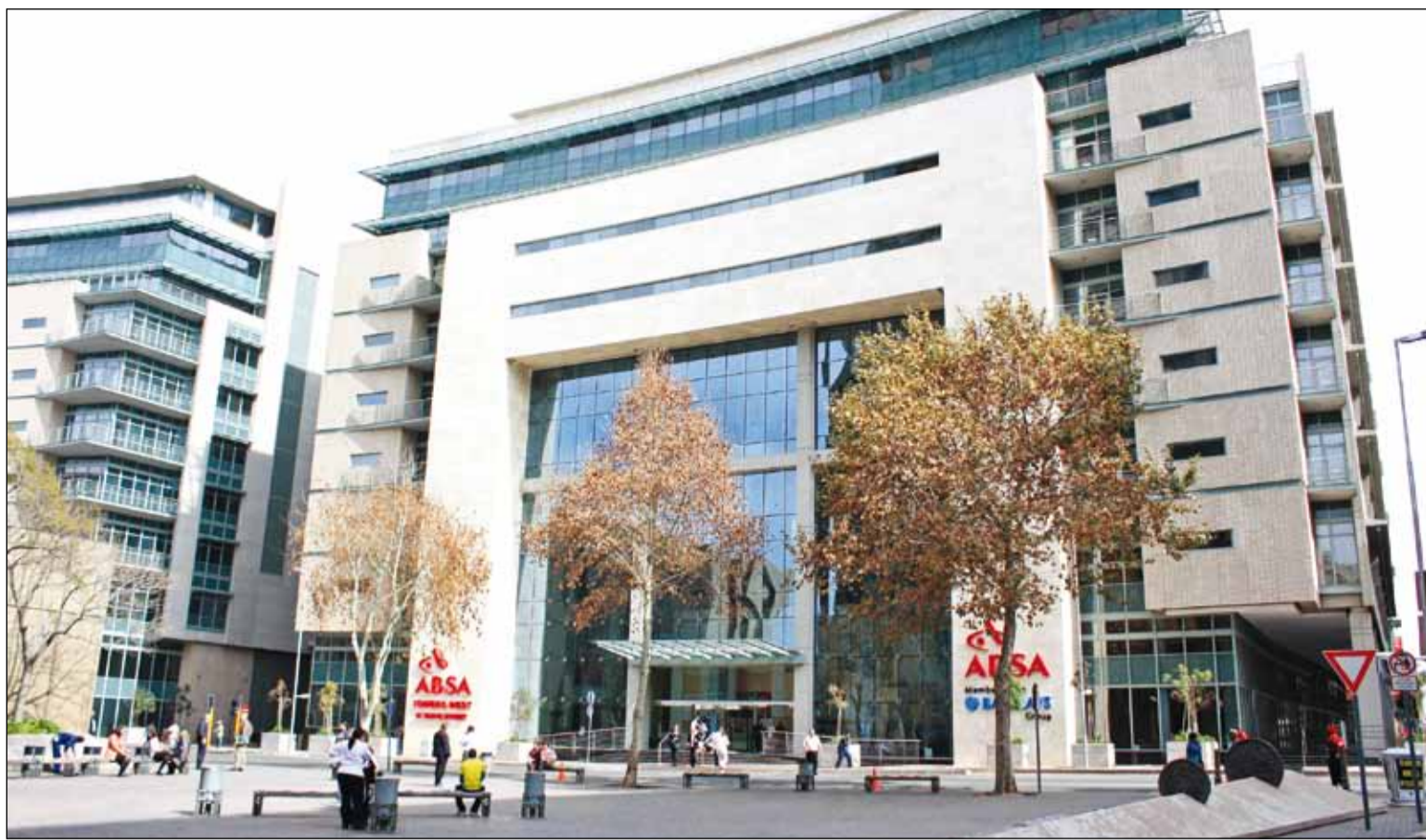
A front view of the energy efficient Absa Towers West (ATW) in the Johannesburg Central Business District.
