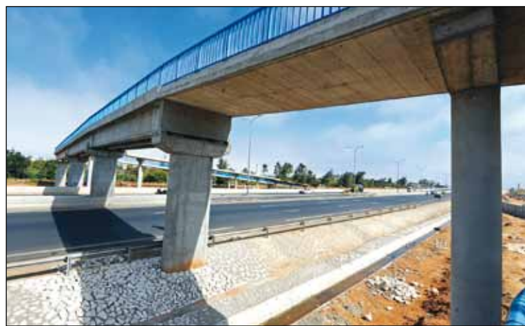
Major new roads and highways are being constructed throughout Senegal.
