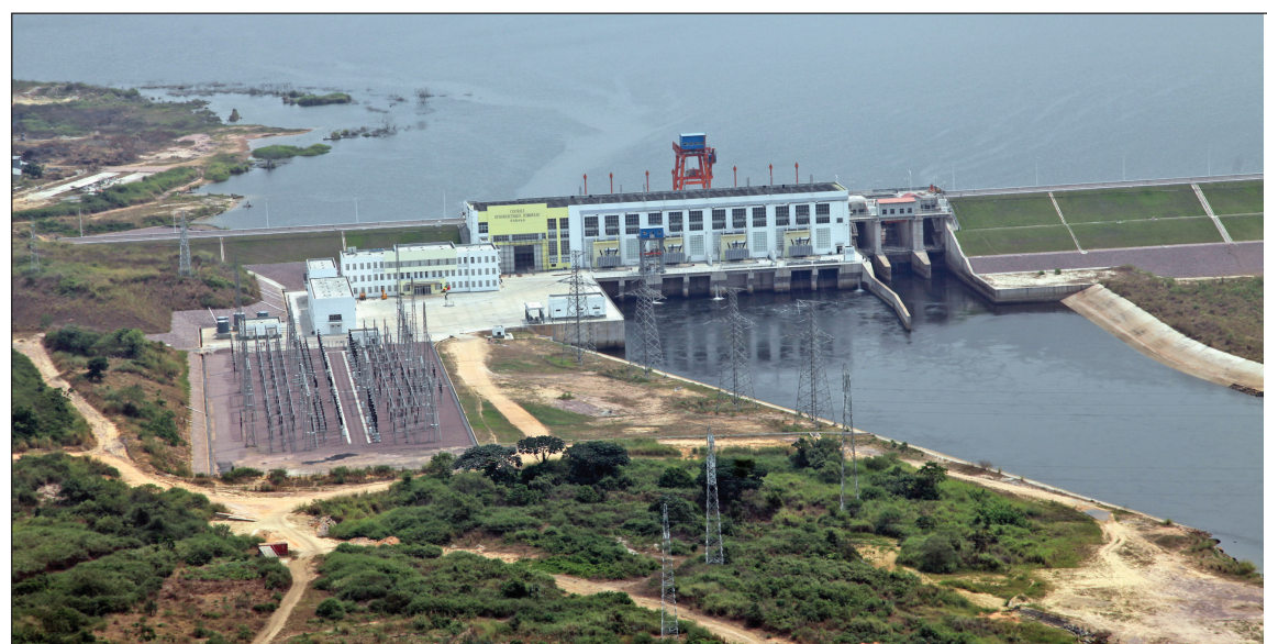
Imboulou Hydroelectric Power Plant.
